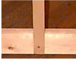
fig. 3: bottom brace with chiseled center support recess
