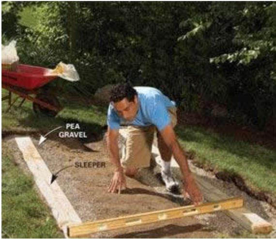
PHOTO 1: LEVEL THE SLEEPERS
