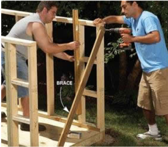
PHOTO 3: ERECT THE WALLS
