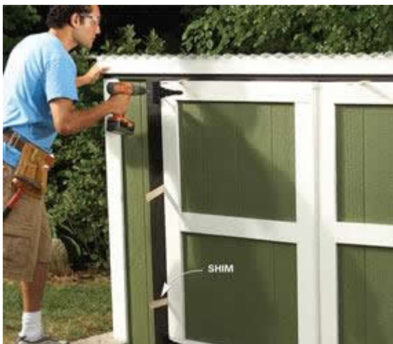
PHOTO 9: HANG THE DOORS
