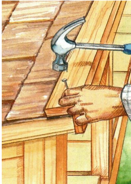
Cover the shingle ends at the top edge of the roof with a 1 × roof cap.
