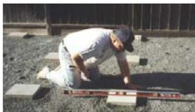
5. To level the blocks, lay them down inside the string perimeter. By using either of the methods outlined above you can square their position properly.
