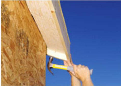
You can also install an overhang on the sides that protects the siding. Add a fascia and soffit, and rake board to the eaves. (Fig. 9)
