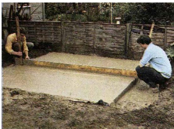
Tamping down the concrete
